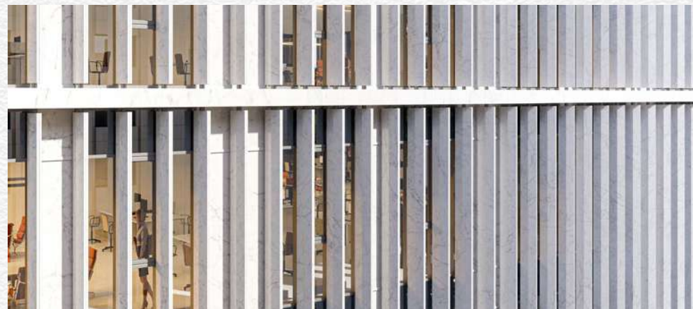
SYGGROU AVENUE 97 OFFICE BUILDING, ATHENS
